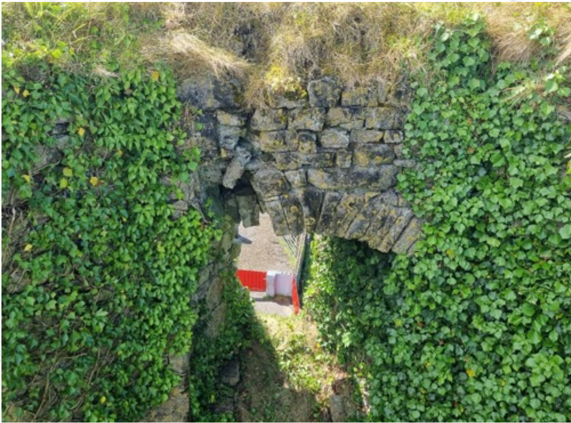
Face of wall showing missing stone voussoirs
