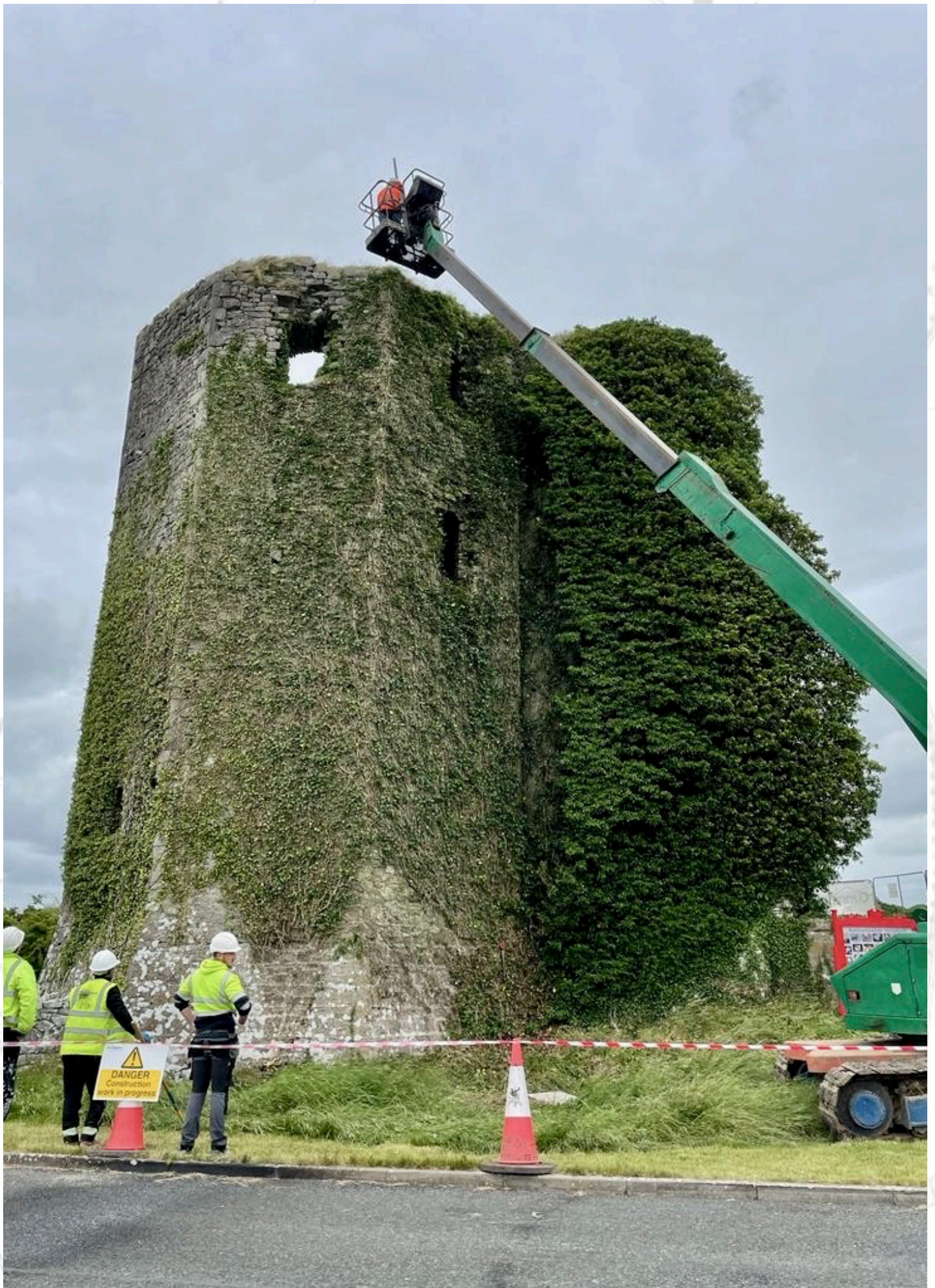
works beginning on the removal of ivy from southwest tower
