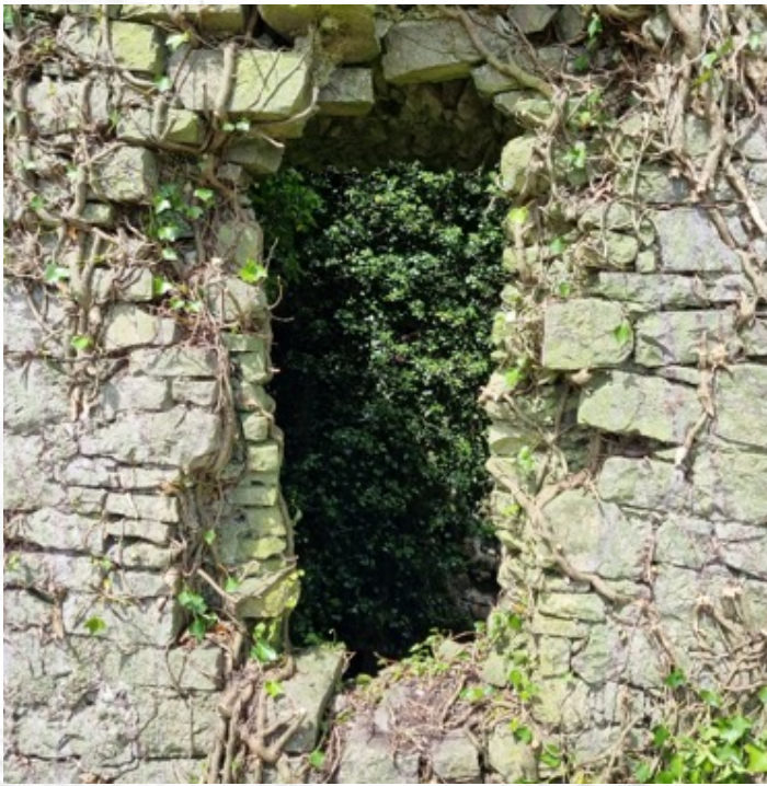
Loose stone around window openings
